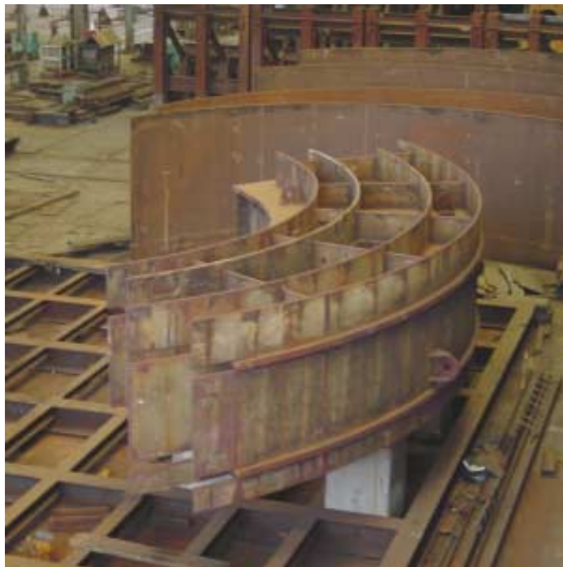
Quadrant View of the Third Layer of the Reactor Pedestal
